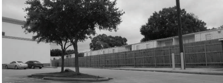
Pedestrian Access Barrier: Fence
