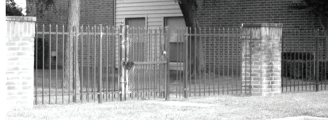
Pedestrian Access Barrier: Fence and Locked Gate
