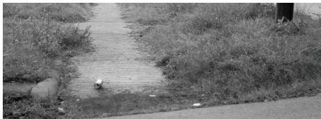
Pedestrian Access Barrier: Poor Sidewalk Condition
